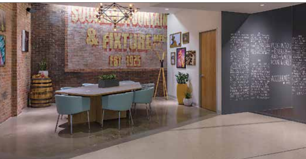
The existing terrazzo was repaired and refinished in this small meeting area.
